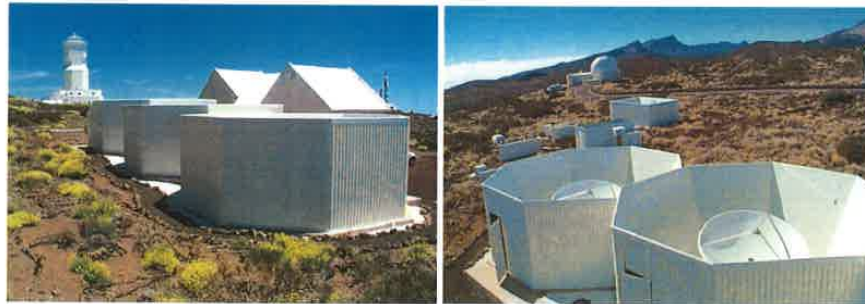
Former VSA enclosures
